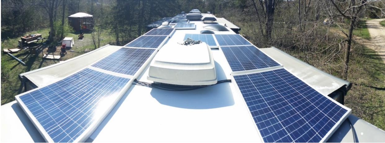
Figure 2. Standing at the rear looking forward. Cables visible routed under and behind the 3rd air conditioner. Dirty rag on top. More wire ties needed.
