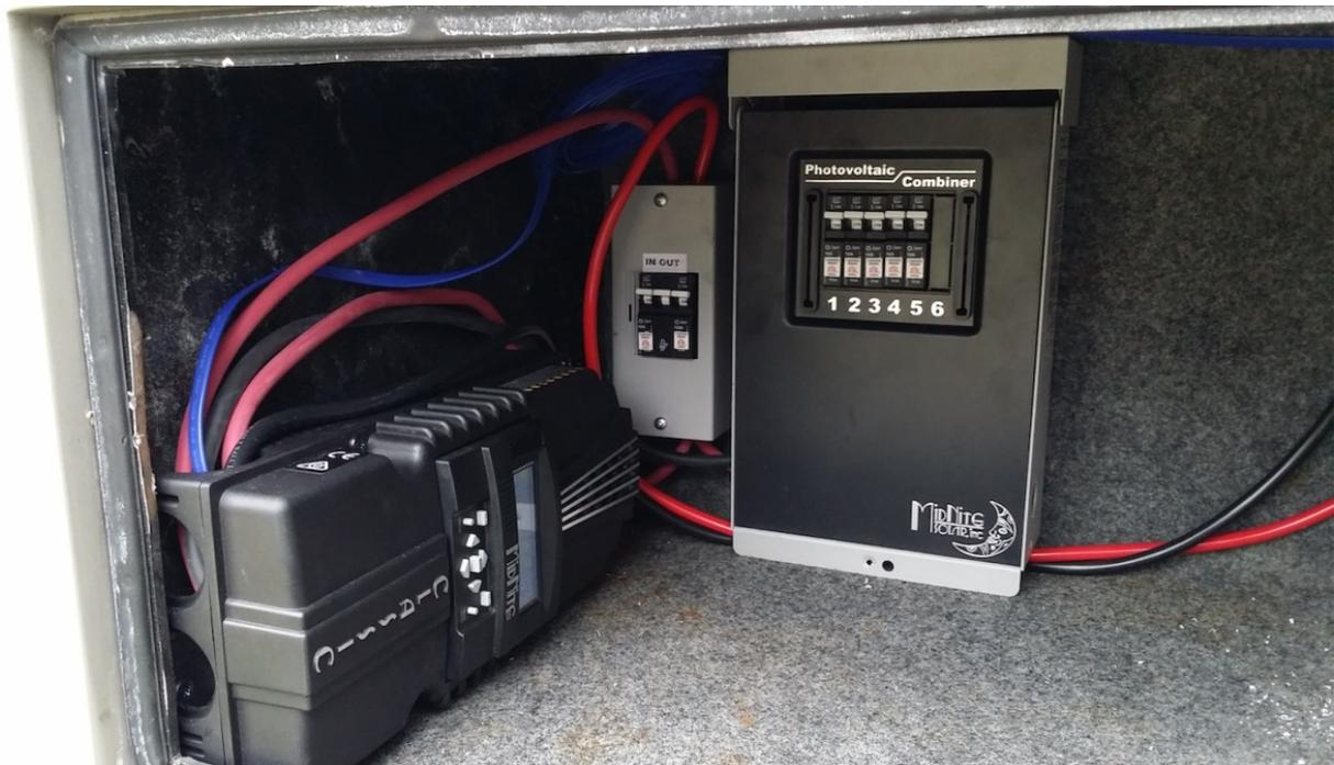
Figure 3. From left to right, charge controller, baby box, combiner box. This is the rearmost storage bay on the curb side of the RV adjacent to the engine.
